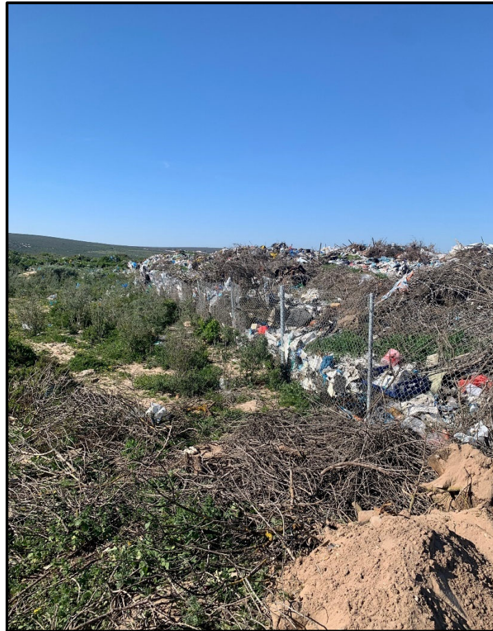
Figure 2-21: Eland's Bay Landfill operations
