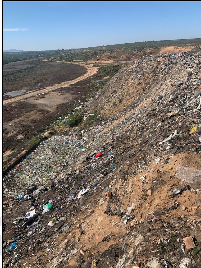
Figure 2-19: Lambert's Bay Landfill problematic steep side slope
